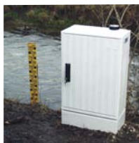
protection housing with puck antenna, modem inside
