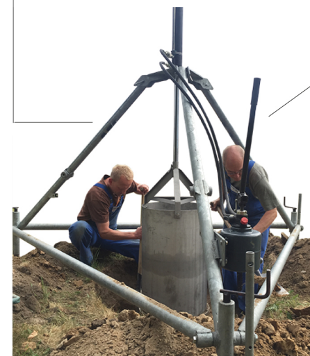
Excavation undisturbed soil monoliths Extended service UGT GmbH
