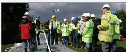
CMT Installation and training as part of a “Multilevel Course” given by the University of Cranfield at Silsoe, U.K., in conjunction with Waterra (UK), British Geological Survey & Norwest Holst.
